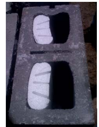
Insulation inserts within CMUs - No Credit allowed in R-Value Method (Use U-Factor Alternative)
